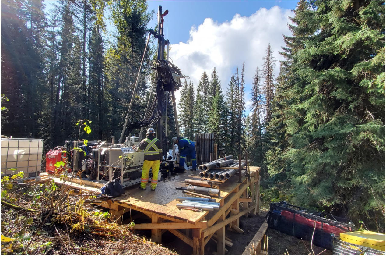
Image 1: Sonic Infrastructure Geotechnical Drilling Underway Within WSF Area
